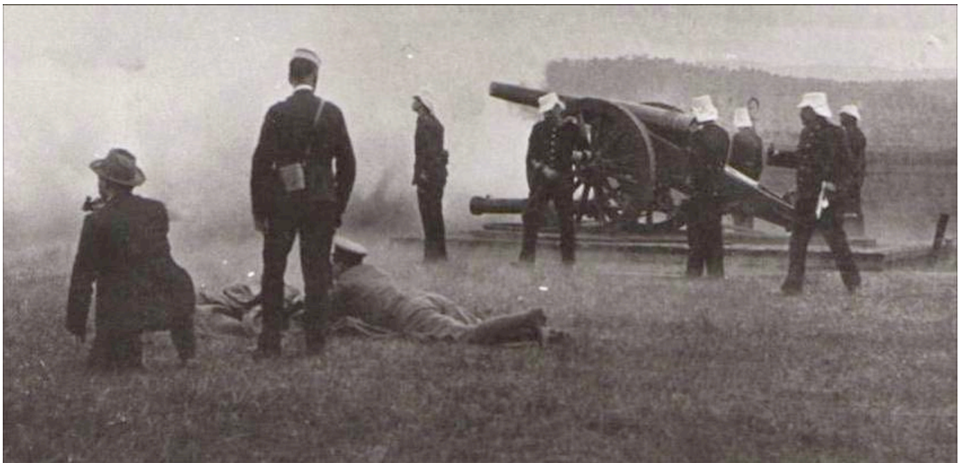
The below image shows the Armstrong 40 Pounder on its Siege Platform at the Ross Easter Encampment. The wooden platform and recoil cylinder are apparent as the gun is in full recoil having just fired.
